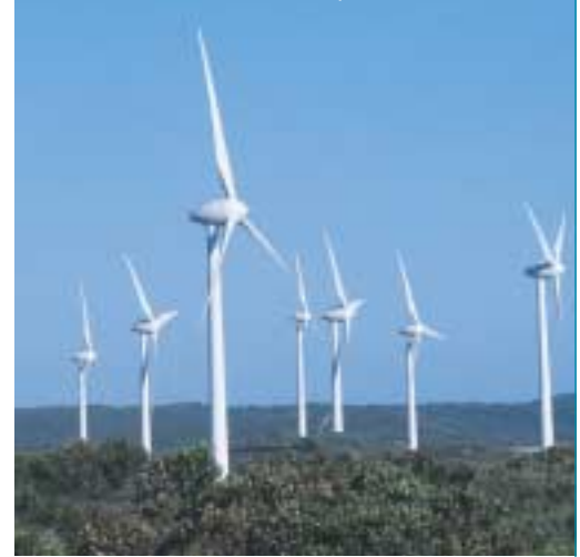
The Albany Wind Farm. Picture courtesy of Western Power
